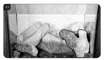
7.8 Use some of the Embaglow provided and cover the ports in the burner tray with a liberal amount of fibres. Use a small piece in front of the log on the left hand side and a long strip in front of log B, see Diagram 12.
