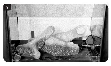
7.6 Log C rests on the cutout on Log E and is pushed up to the side and rear of the firebox, see Diagram 10.
