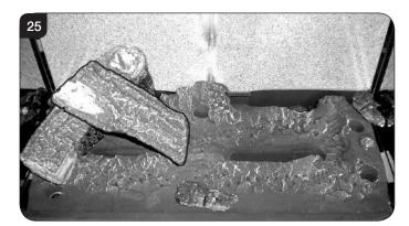
7.21 Place Log C on the right hand side of the burner. There is a hole on the underside of Log C which fits over the raised stud on the right of the burner. The back of the log should rest flush against the back panel, see Diagram 26.
