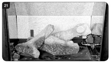
9.6 Log C rests on the cutout on Log E and is pushed up to the side and rear of the firebox, see Diagram 22.
