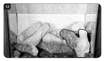
7.8 Sparingly spread an amount of the Embaglow fibres provided, covering the ports in the burner tray. Use a small piece in front of the log on the left hand side and a long strip in front of log B, see Diagram 13.
