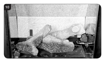
7.6 Log C rests on the cutout on Log E and is pushed up to the side and rear of the firebox, see Diagram 11.
