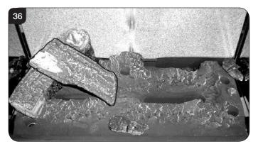
9.21 Place Log C on the right hand side of the burner. There is a hole on the underside of Log C which fits over the raised stud on the right of the burner. The back of the log should rest flush against the back panel, see Diagram 37.
