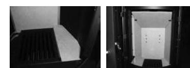
Outer top baffle brick 11 (smallest straight edge resting on top edge of rear brick) fitted and supported with two side pins.
