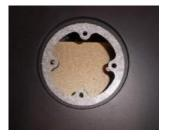
Place the flue collar gaskets on the outlet to be used.
