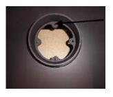
Wind the four M6 studs supplied into the fixing holes in the flue collar until finger tight. Place the flue collar onto the stove and tighten using the supplied washers and nuts from inside the stove.
