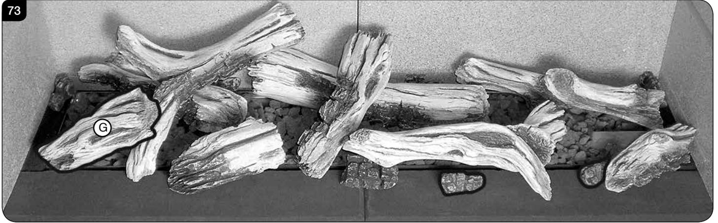
13.16 Once all the logs are in place, spread the remaining lava rock across the front and side liners, see Diagram 74.
