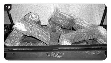
7.17 Once the logs are in place sparingly spread an amount of the Embaglow fibres provided on the sections highlighted, see Diagram 20.
