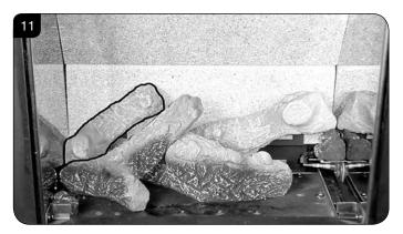
8.7 Place the pointed bottom of log D into the corner of the burner tray and rest on the location stud in log B, see Diagram 12.
