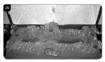
7.19 Place Log D on the left hand side of the burner. There is a hole on the underside of Log D which fits over the raised stud on the left of the burner. The back of the log should rest flat against the back panel, see Diagram 27.
