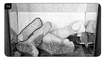
7.7 Place the pointed bottom of log D into the corner of the burner tray and rest on the location stud on log B, see Diagram 15.
