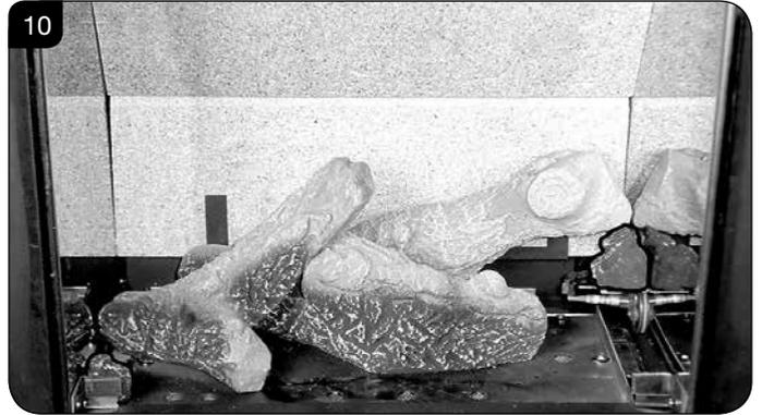
8.6 Log C rests on the cutout on Log E and is pushed up to the side and rear of the firebox, see Diagram 11.
