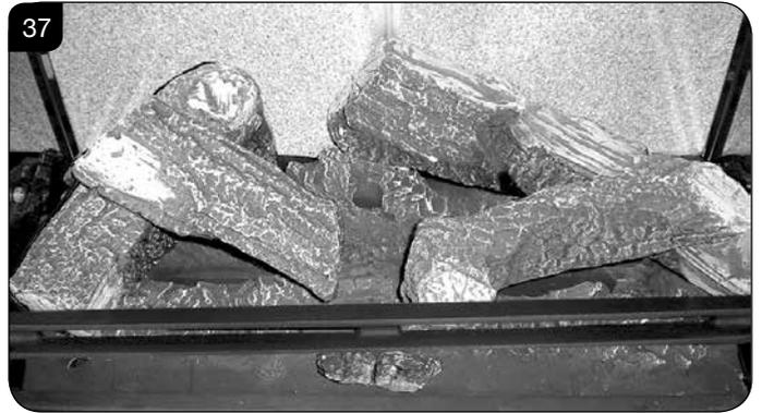
7.24 Once the logs are in place use some of the Embaglow wire wool provided and cover the ports in the burner tray with a liberal amount of fibres, in the highlighted areas shown in Diagram 38.
