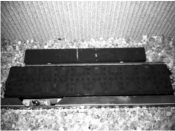
The granules can then be spread around the fire tray and behind the fibre strip packing it to ensure the strip cannot move
