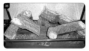
8.21 Once the logs are in place use some of the Embaglow wire wool provided and cover the ports in the burner tray with a liberal amount of fibres, in the highlighted areas shown in Diagram 37.
