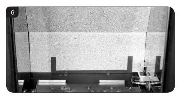
7.2 Place Log A on the higher rear bracket and push up against the back panel, see Diagram 7.
