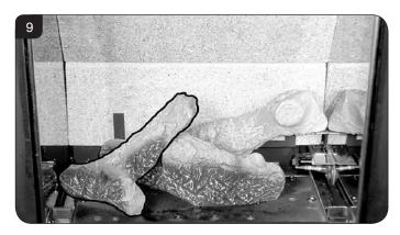
7.5 Place the small Ember at the front left of the firebox, against the rear of the log support bracket to obscure the reflection of the burner screw.
