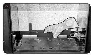
7.3 Place Log B over the two middle studs on the burner tray, see Diagram 6.
