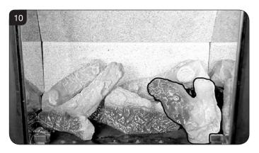
7.8 Use some of the Embaglow provided and cover the ports in the burner tray with a liberal amount of fibres. Use a small piece in front of the log on the left hand side and a long strip in front of log B, see Diagram 11.
