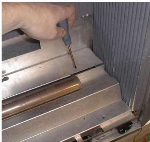
**6.4** Remove the appropriate knockout in the side or the rear of the fire box for the gas supply pipe and fit the supplied rubber grommet. Make a small incision in the grommet to accept the gas supply pipe.
