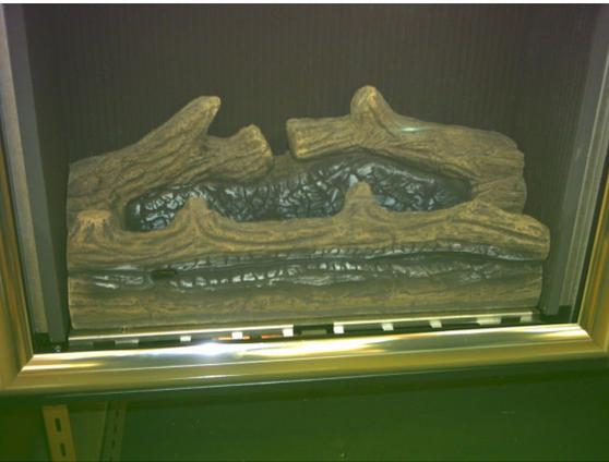
8.1.2 Carefully place the front log piece on the support platform in front of the burner. Ensure that the base of this piece is flat and slowly push back until it touches the protruding ends of
