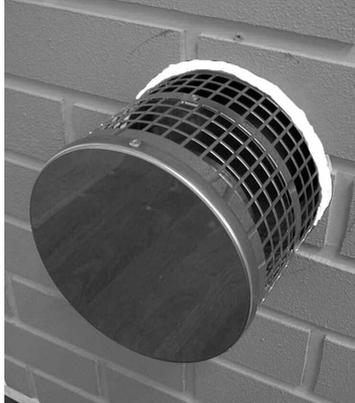
**NOTE:** In England & Wales, the building regulations require that a terminal guard should be fitted if the terminal could come into contact with people near the building or be subject to damage. BFM Europe Ltd. also recommend the fitting of a flue terminal guard where regulations do not demand that it be fitted. A suitable flue terminal guard is supplied with the appliance.
