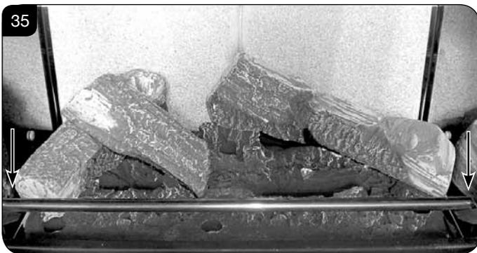
8.20 Place Log A across Log C. There is a hole on the underside of Log A which fits over the raised stud on Log C to secure in place. The small cut out on the left side of the log rests onto the log guard, see Diagram 36.
