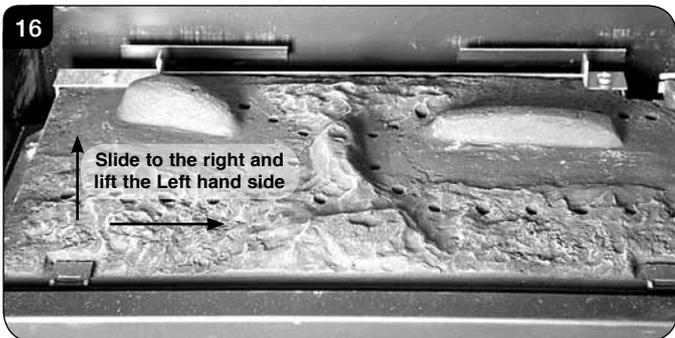
6.5 Slide the burner back to the left and out of its location. **IMPORTANT: Take care when removing the burner not to damage the ceramic pad with the pilot unit attached.**
